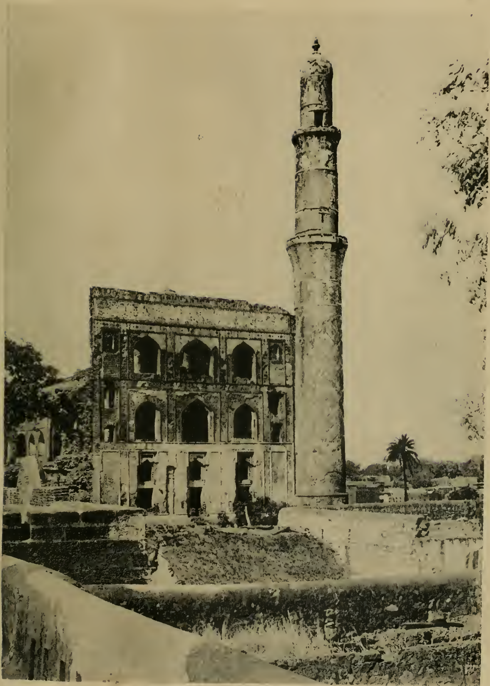
BIDAR MADRASA: NORTHERN END OF EAST FAÇADE.
