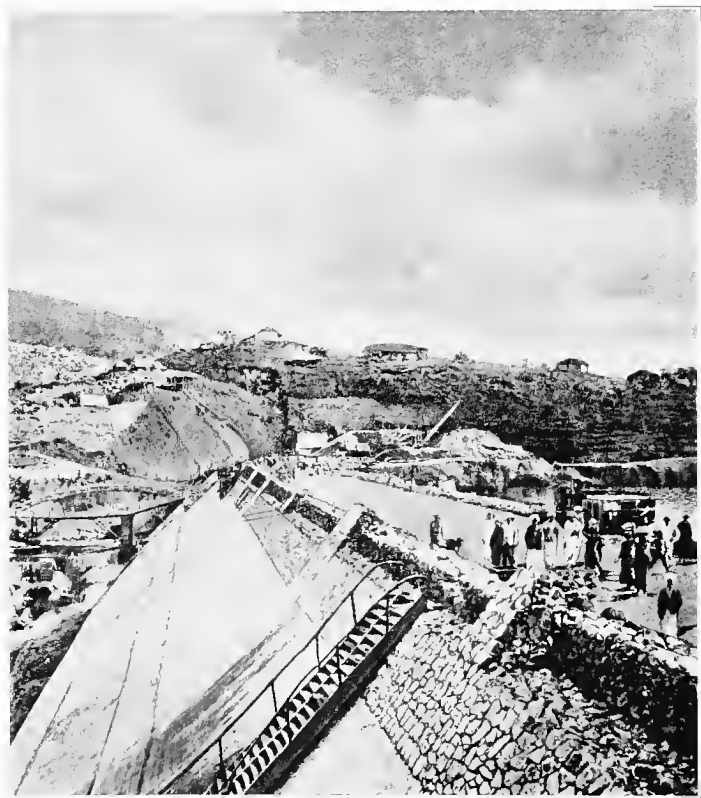
Fig. 71. Periyar dam during construction.
